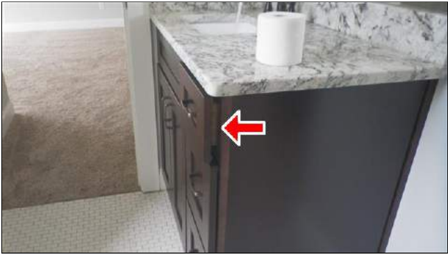
(5) Inside the 2nd floor right side Jack & Jill bathroom, one of the cabinet doors has a loose hinge.
