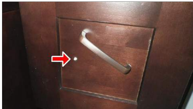
(4) Inside the 2nd floor right side Jack & Jill bathroom, one of the drawers does not fully close.
